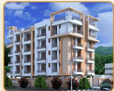
Dhairya Nikunj Sunderpur, Varanasi
